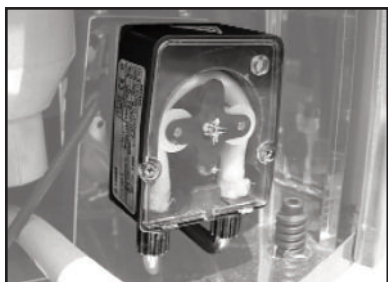
Built-in detergent and rinse chemical pumps.
